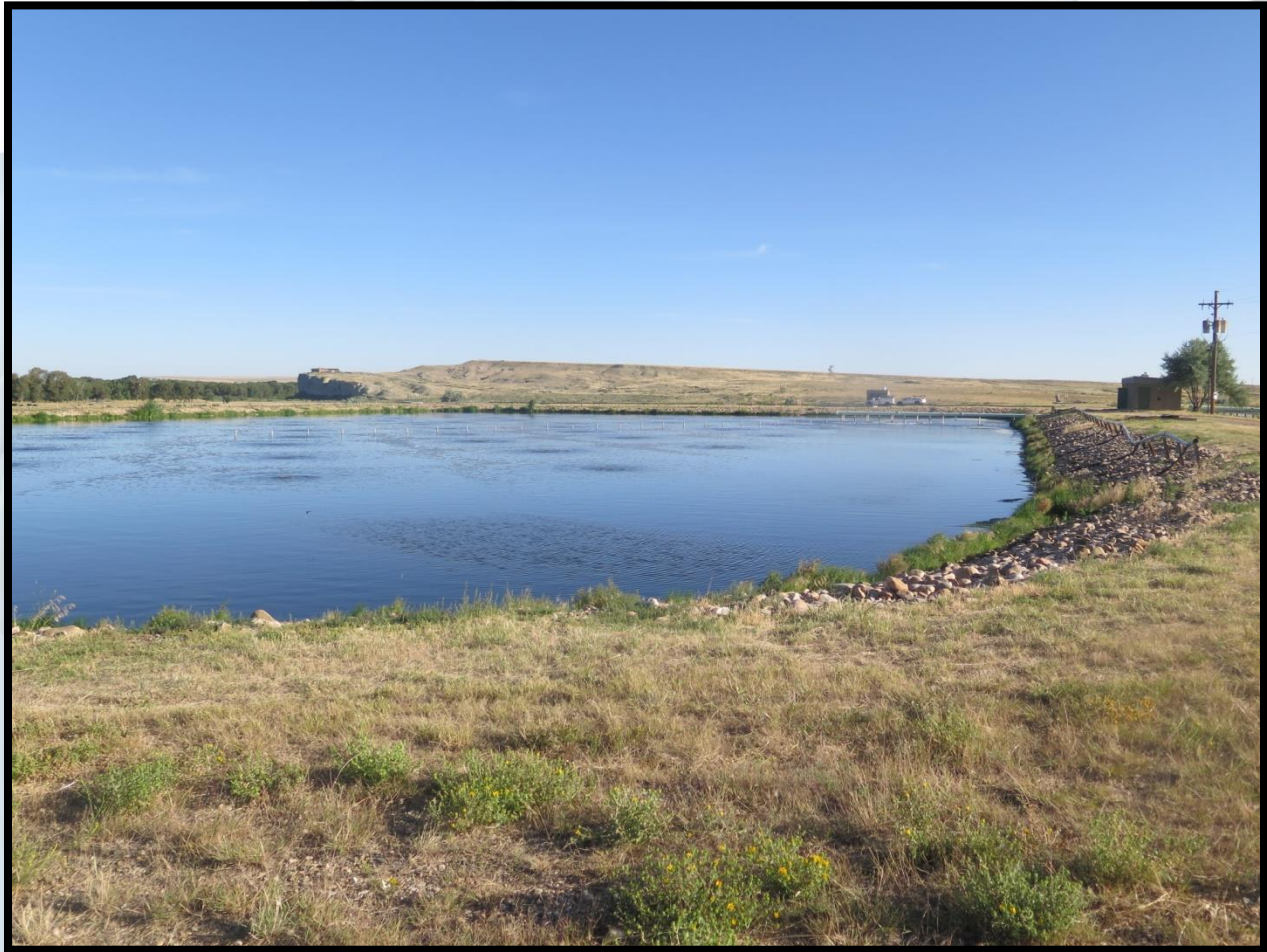
Wastewater Treatment Lagoon
