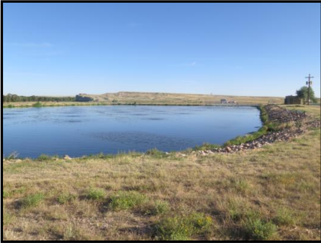
Wastewater Treatment Lagoon
