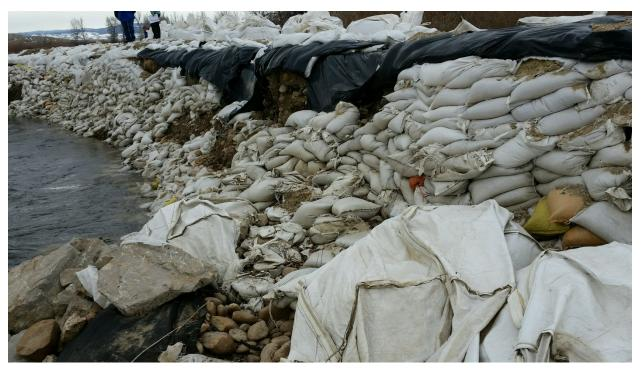
Photo No. 4 – View of the upstream face of the embankment, from near the upstream culvert, looking upstream. Note the vertical embankment face, deteriorating sandbags, and exp0sed embankment material.
